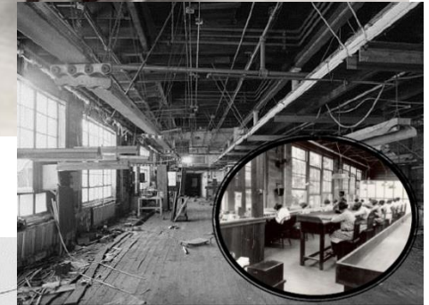
US Radium Paint Application Building, 2nd floor, 1998 Insert: Dial Painters in same room, 1922
